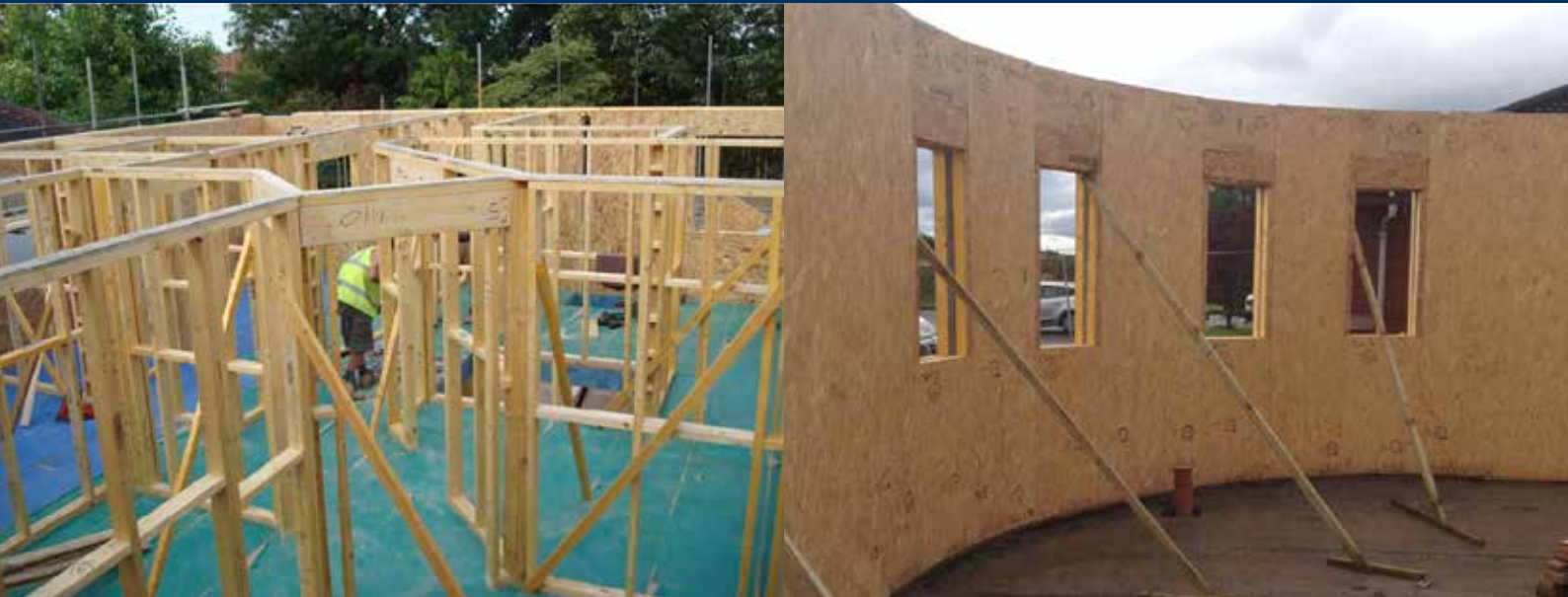
95mm x 45mm timber studwork is used to construct internal Walls Sips Eco panels can easily be used to create curved walls
