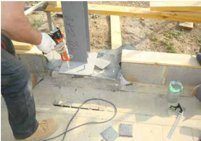
With the steel base plate in position, holes are drilled into the padstone and then filled with resin.
