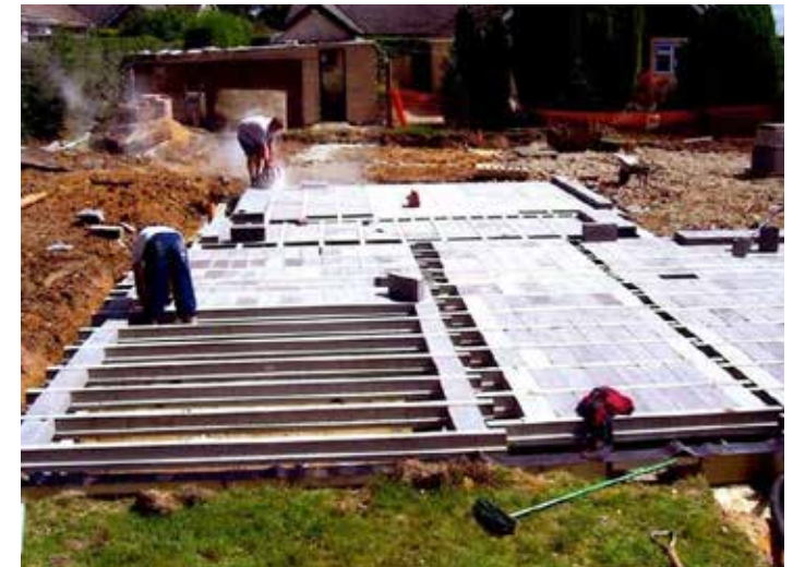
Ground floor being laid
