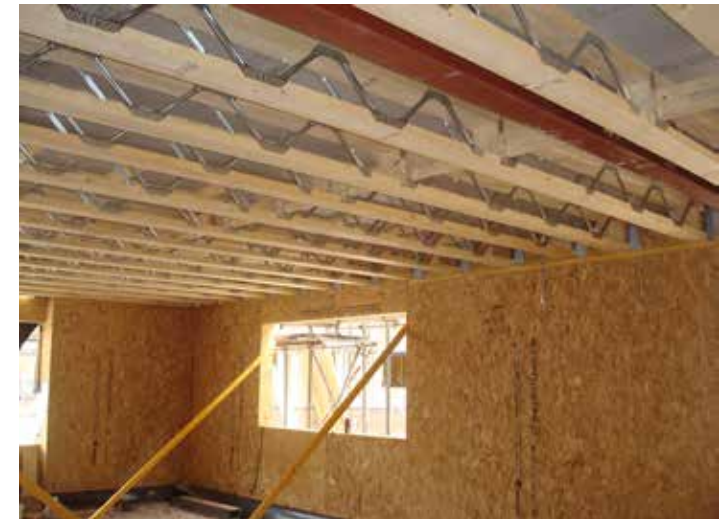
First floor joists fitted
