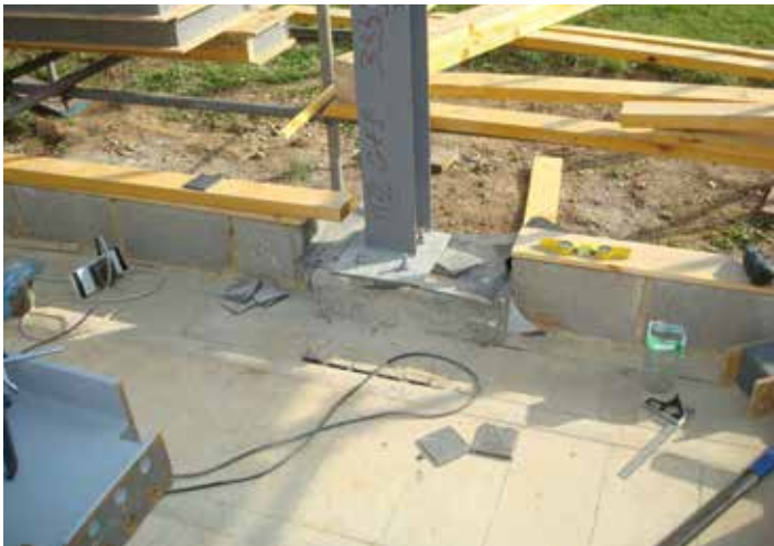
Nuts are screwed tightly with a wrench onto the bolts.
