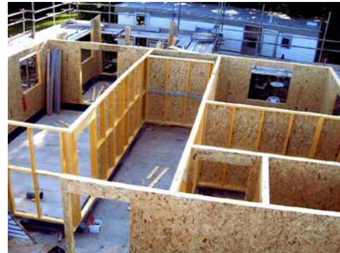
Ground floor walls being erected
