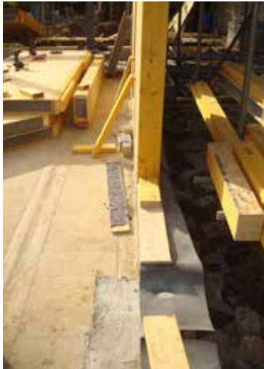
Upstands must be dense concrete blocks or concrete. These are built to the same height as the finished floor for external and internal walls.
