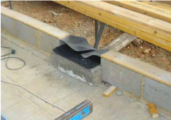
A concrete padstone is cast and set 80mm lower than the finished floor level. A DPC is fitted and then the steel post base plate is positioned.
