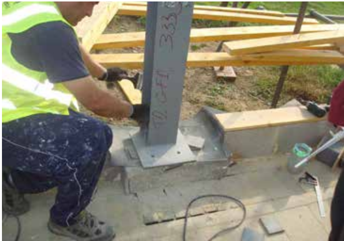
The steel is located in accordance with the FLP. It can be positioned vertically plumb by using steel shims.
