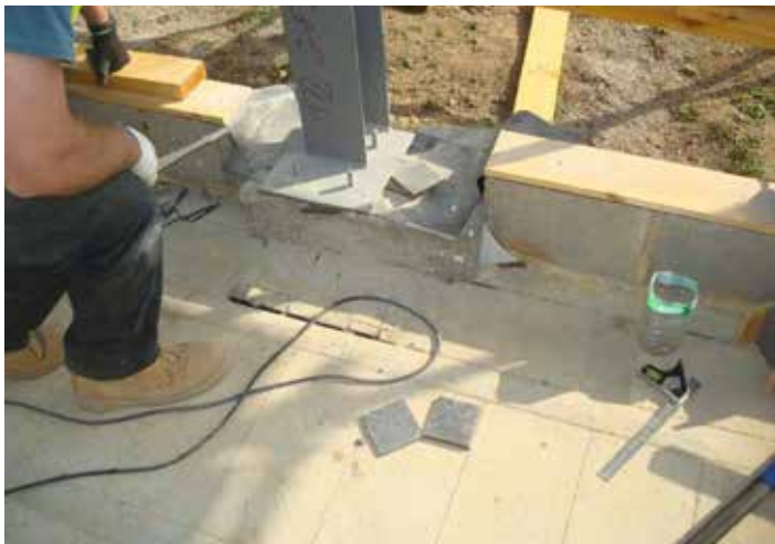
Bolts are slotted into the holes and left to set in position in the resin.
